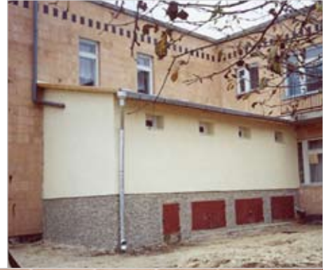
Indoor ecological toilet building for the school of Gozhuli
