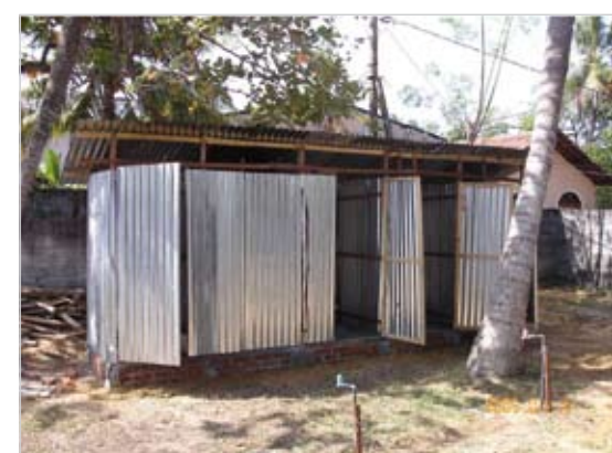
Simple construction of a pit latrine in Sri Lanka
