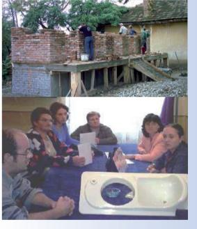
Construction of the toilet building with local material
