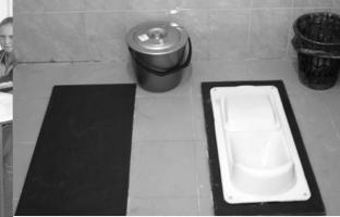
Restroom with the squatting slab on the right. When the right faeces chamber is full, the slab has to be switched to the left side and the right place will be closed
