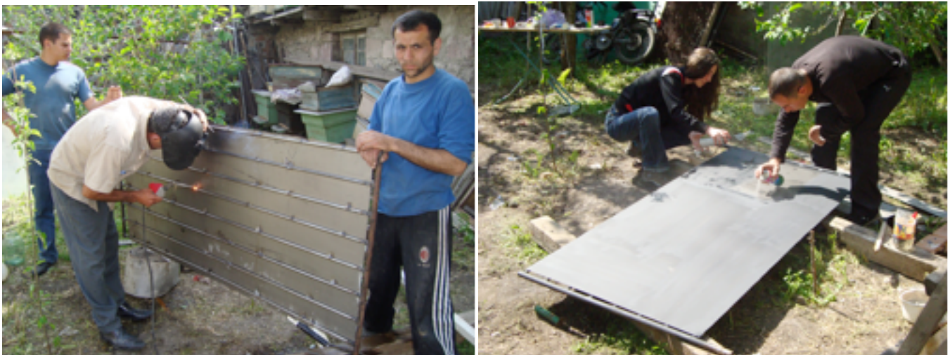
construction and painting of the metal flat-plate collector
