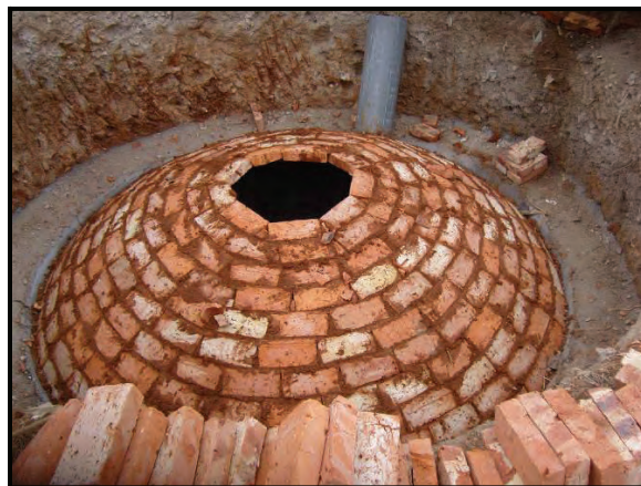
A biogas tank under construction
