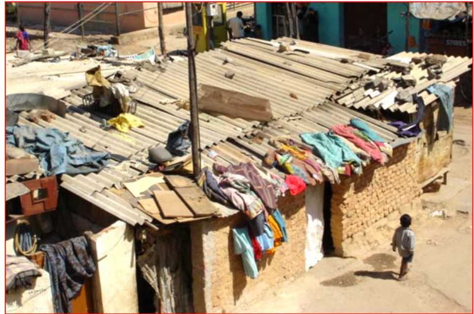
Typical asbestos cement (AC) roofing in the countries where asbestos is not phased out
