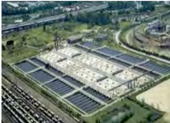
View on a huge technical wastewater treatment plant in Hamburg Source: http://www.vdi.de/2151.0.html
