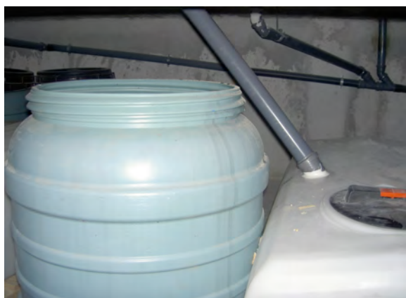
Urine and the faecal matter of the urine diverting dry toilet are separated and collected in different containers, and treated for safe reuse in the garden of the community centre in Sulitsa
