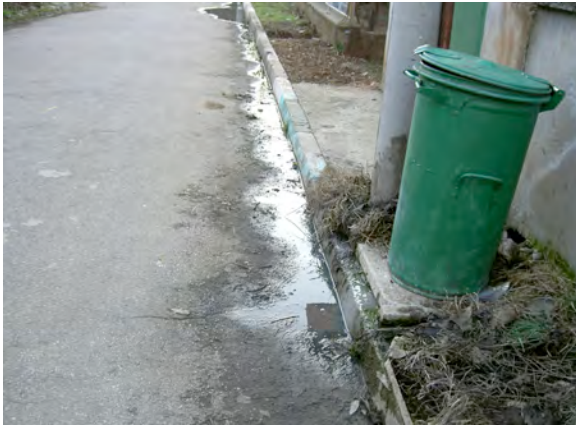
A street contaminated by wastewater from overflowing septic tanks
