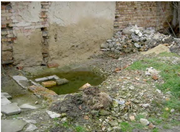
A soak away pit filled with wastewater
