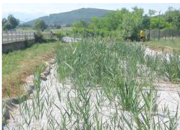
Soil filter with planted reed in Vidrare Photo: Bistra Mihaylova
