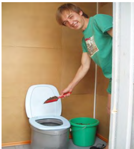
Toilet flushing after use in case of a urine diverting dry toilet in Ukraine
