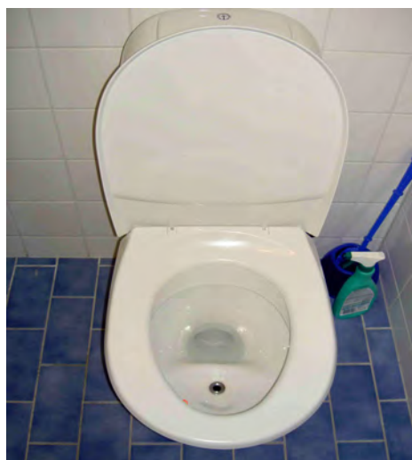
Urine diverting toilet with water flush
