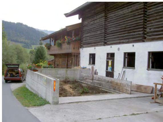
Manure should be stored on a closed concrete platform
