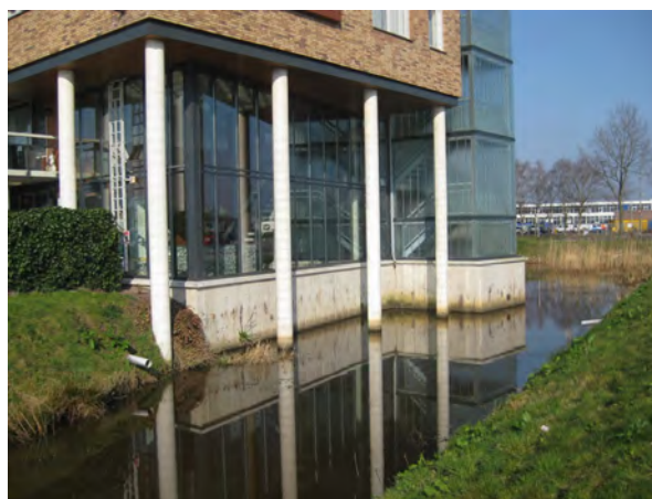
Artificial water course/trench for rainwater retention
