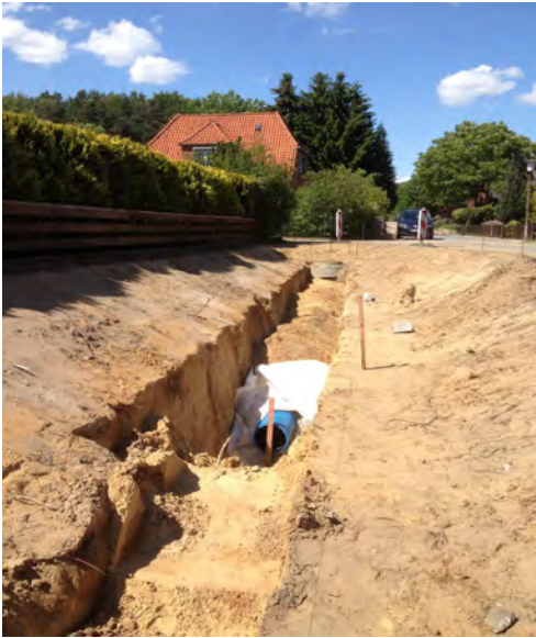
Rigole infiltration system in construction Photo: Arnd Wendland
