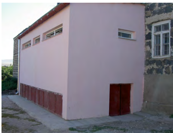
Exterior of a UDDT facility attached to a school
