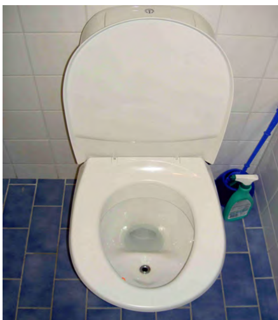
Urine diverting toilet with water flush
