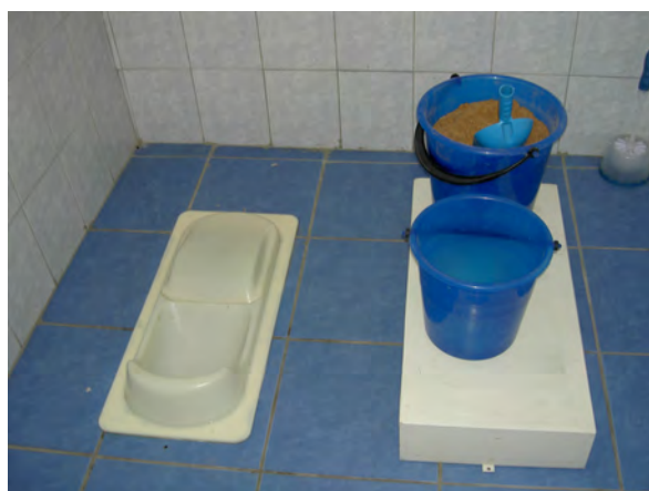
Interior of the toilet cabin
