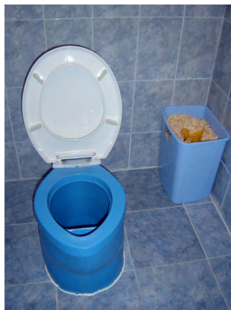
Interior of an Ecosan toilet, toilet (UDDT), constructed inside of a house in Bulgaria. Photo Earth Forever
