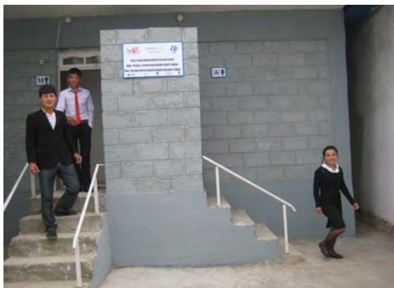
Separated toilet facilities for boys and girls
