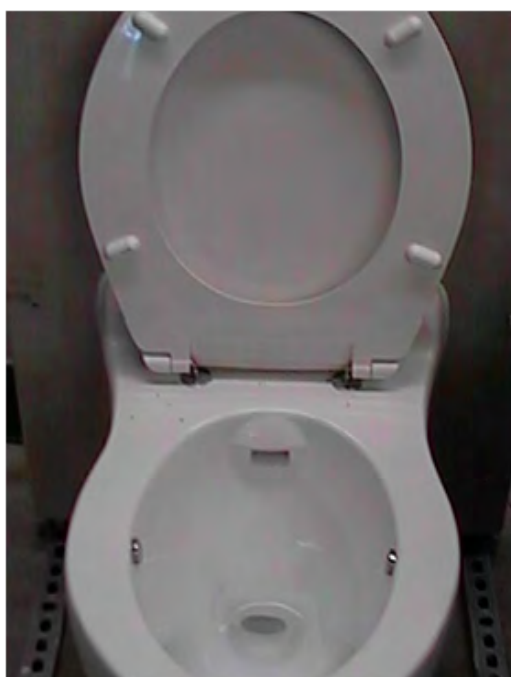
Vacuum toilet using one liter per flush
