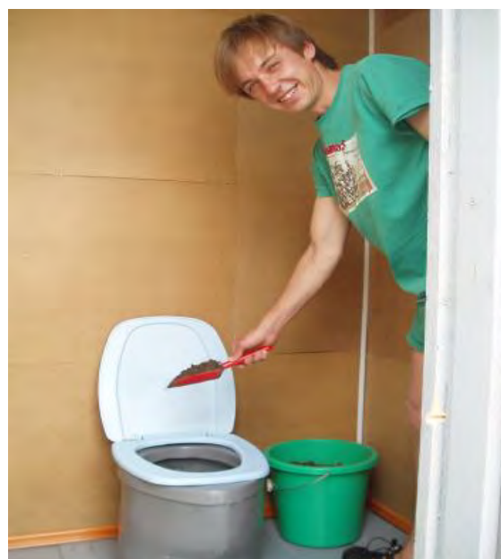
Toilet flushing after use in case of a urine diverting dry toilet (UDDT) in Ukraine
