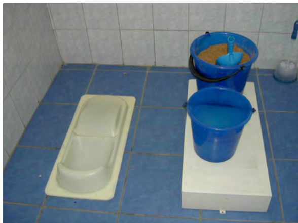
Interior of the toilet cabin
