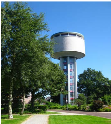
A water tower maintaining an appropriate pressure day and night
