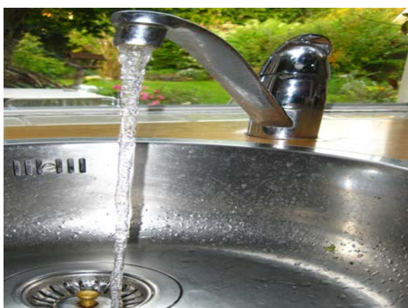
After passing kilometers of pipes, the water quality at household level could be decreased and is often not known
