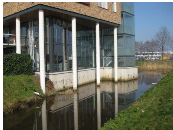
Artificial water course/trench for rainwater retention
