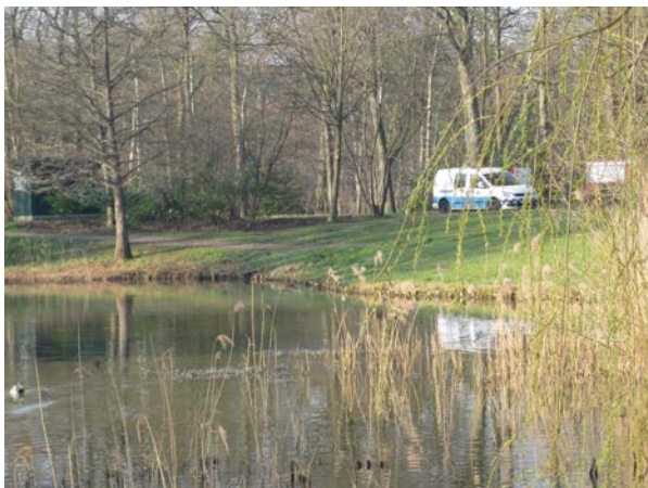
Artificial retention pond
