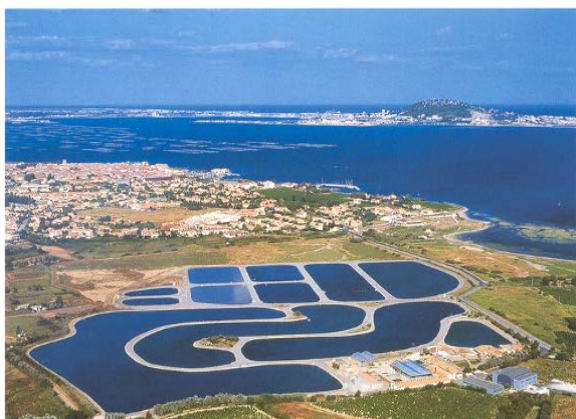
Pond system in Meze, France (Photo: Francois Brissaud)
