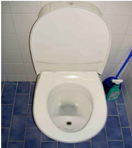
Urine diverting toilet with water flush
