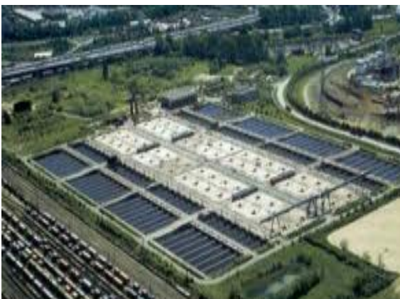
View on a huge technical wastewater treatment plant in Hamburg
