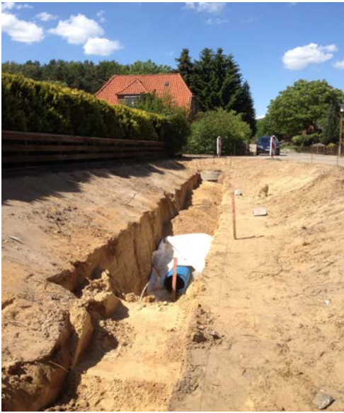
Rigole infiltration system in construction Photo: Arnd Wendland
