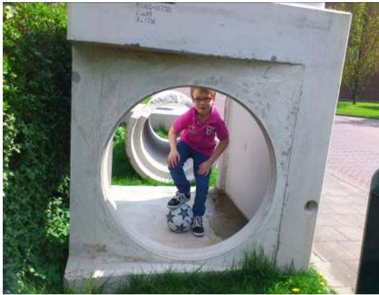
Wastewater collection pipe including a man hole which will be put underground
