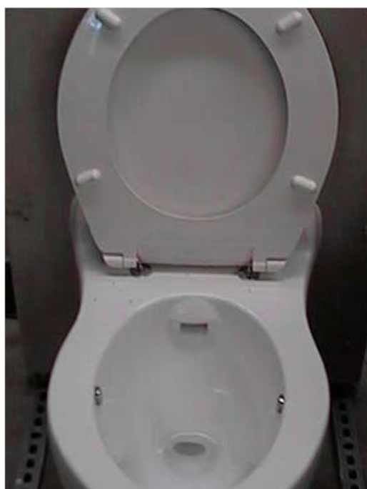
Vacuum toilet using one liter per flush
