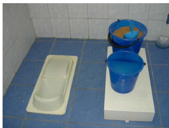
Interior of a UDDT cabin
