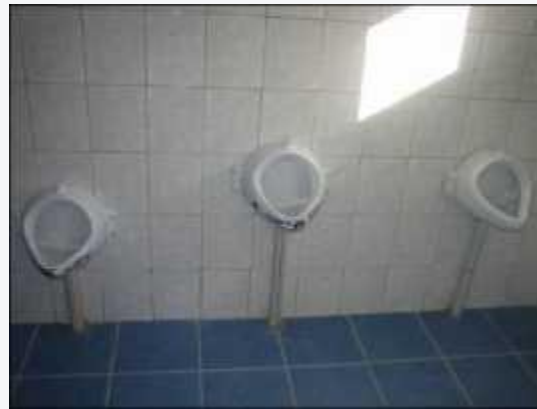
Waterless urinals at different heights
