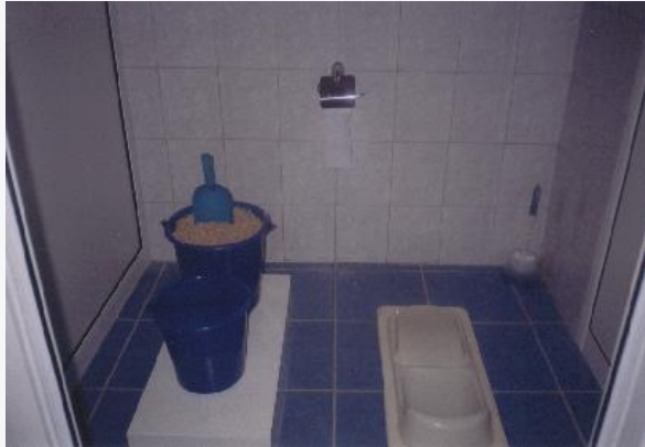
Squatting toilet with urine diversion
