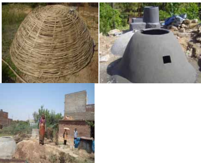
Pictures: Bamboo basket as reinforcement for cement dome for biogas, biogas plants under construction, finished biogas plant covered with soil
